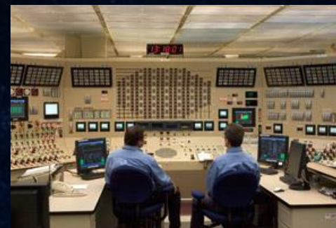
Fire Control Room
